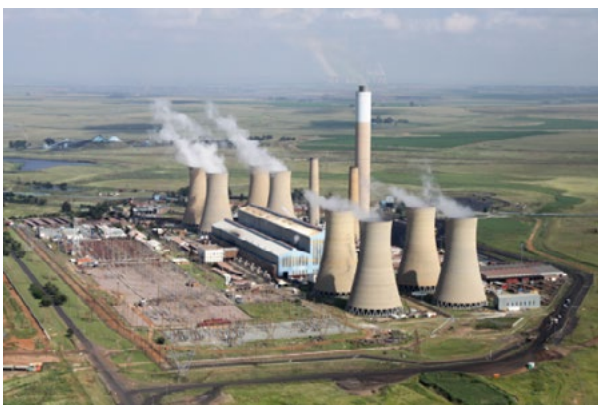
Aerial view of Komati Power Station
